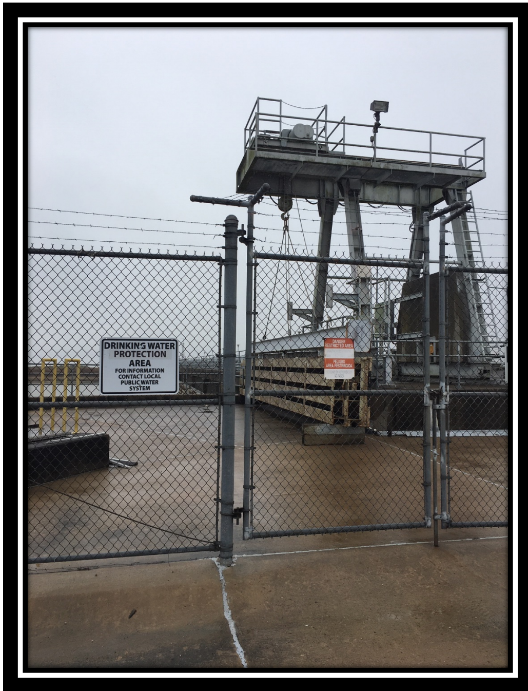
Figure 4: Source Water Protection Signage at Palmetto Bend Dam.
